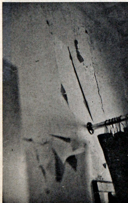
Paint peels off a bathroom wall.
